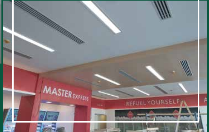
Master Express Lighting Project
